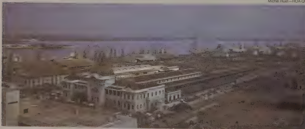
The port and railway complex at Maputo, Mozambique.
